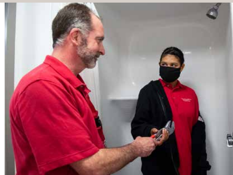
Northeastern University plumber Mike Frost hands Olivia Genera, a Madison Park Technical school student who is working as a plumbing apprentice on campus at Northeastern University, a wrench as she works on fixing a shower in the East Village dormitory. Photo by Alyssa Stone/Northeastern University
